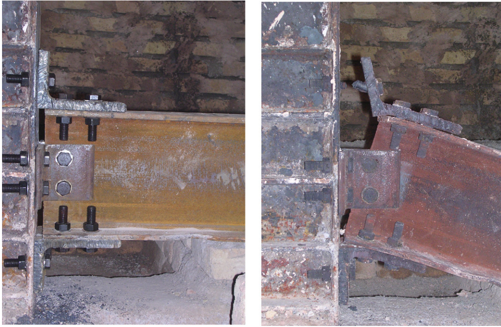
Fig. 17. Specimen 5, failure mode I.
